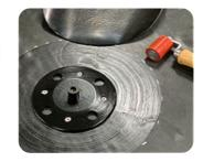
Place the EPDM Covertape (with protective film) over the mounting plate and and draw the edge zone with a crayon. The EPDM covertape can now be incorporated watertight in accordance with the manufacturer's processing instructions. Prime the base plate and the roof covering with an primer. (The EPDM primer has a drying time of approx. 5 minutes)
